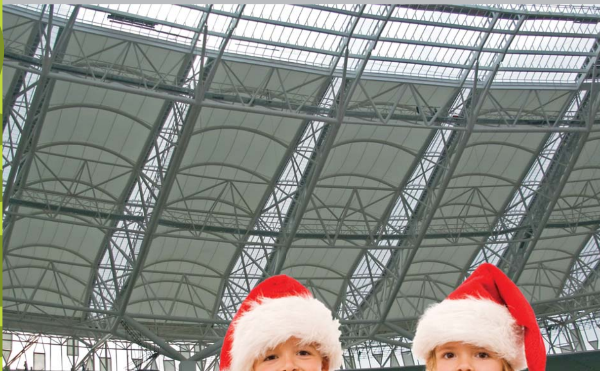
[SUNPAL® skylights installed in Huizhou stadium, China (See article inside).]
